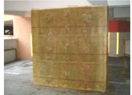
3) Wrapped Column After application of Sand
