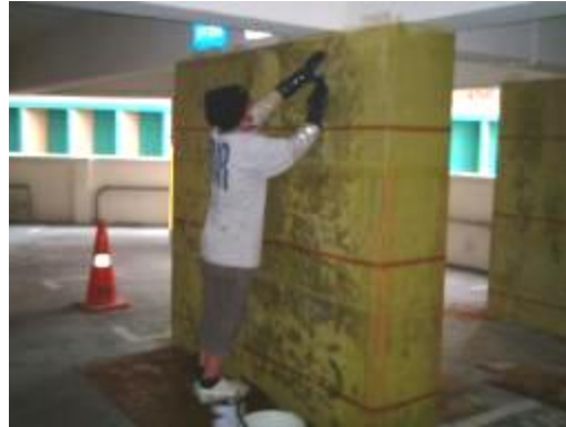
2) Wrapping Work In Progress
