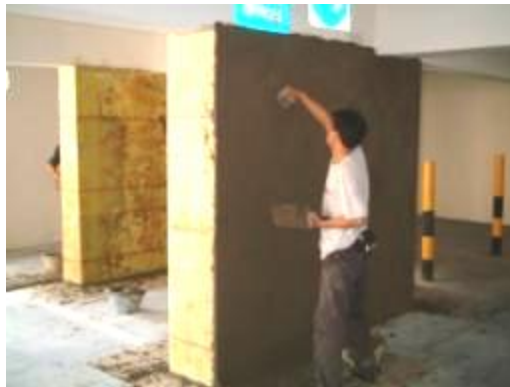
4) Plastering Work In Progress
