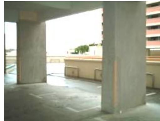
5) Columns Ready for Painting
