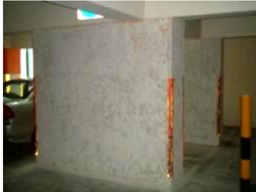
1) Columns After Grinding Ready for Wrapping
